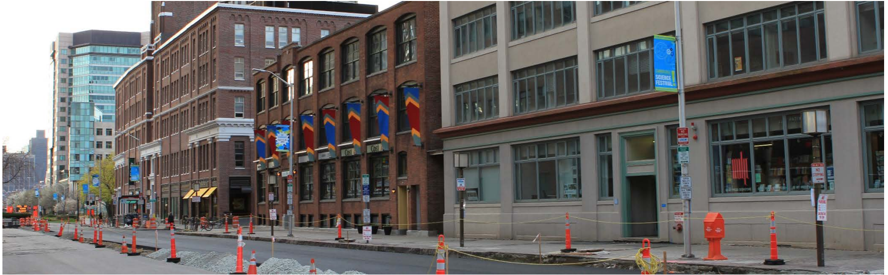
Existing view from looking east down Main Street
